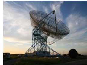
Figure 3. Stanford SRI 45-meter dish at Stanford CA, USA
