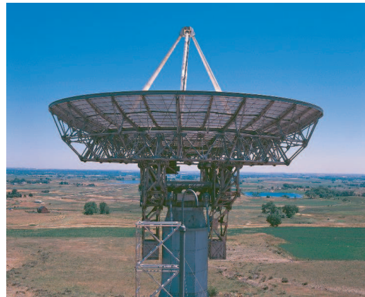
Fig. 4. The 20-meter parabolic antenna of the Institute for Telecommunication Sciences, Table Mountain, Colorado
